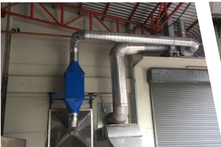
Installation of additional Control Systems and Protections against Odors from the Bread Fermentation Processing
