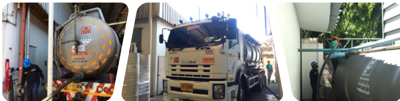
Image of Sludge removal from Wastewater Treatment System
